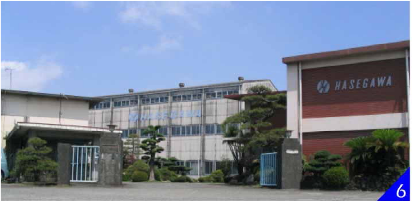
Fig.6 Office(right) Assembling shop(center)
